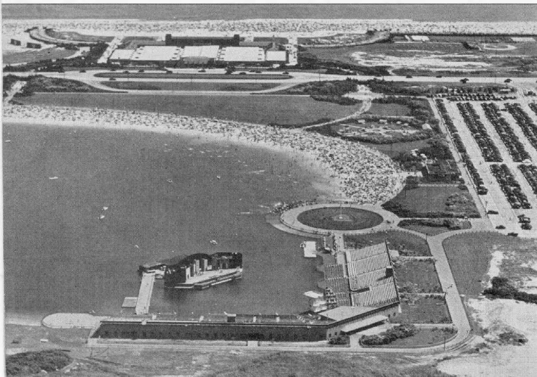
FIGURE 1. View of a portion of Jones Beach, showing the Marine Stadium.
